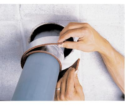
reenterable with no special tools required and are non-flame supporting. Applications include: telephone cable, metal pipe, plastic pipe, conduit, insulated metal pipe and cable trays. They can be used to firestop up to 10 inch (254,0 mm) diameter PVC pipe and are UL-Classified for use on PVC, CPVC, ABS, CCPVC, CCABS, PVDF, FRPP, PP and PB plastic pipe.
