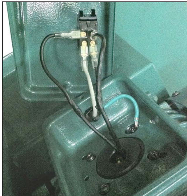
Figure 75. G1029Z2 junction box and switch.
