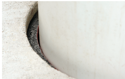
Once installed, wrap strip should be seated slightly below concrete floor surface.
