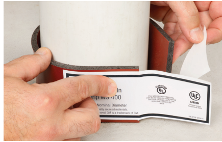
Wrap 3M™ Fire Barrier Tuck-In Wrap Strip around pipe, over floor opening, and adhere label to adjacent side of foam strip.
