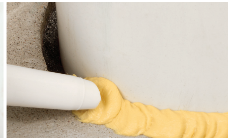
Follow wrap installation with layer of 3M™ Fire Barrier Sealant CP 25 WB+, IC 15 WB+, or 3000 WT to create seal that meets code, fire-rated to 3 hours.
