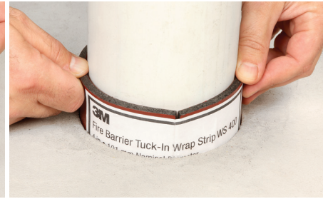
Gently slide wrap strip downward into concrete floor to fill gaps.
